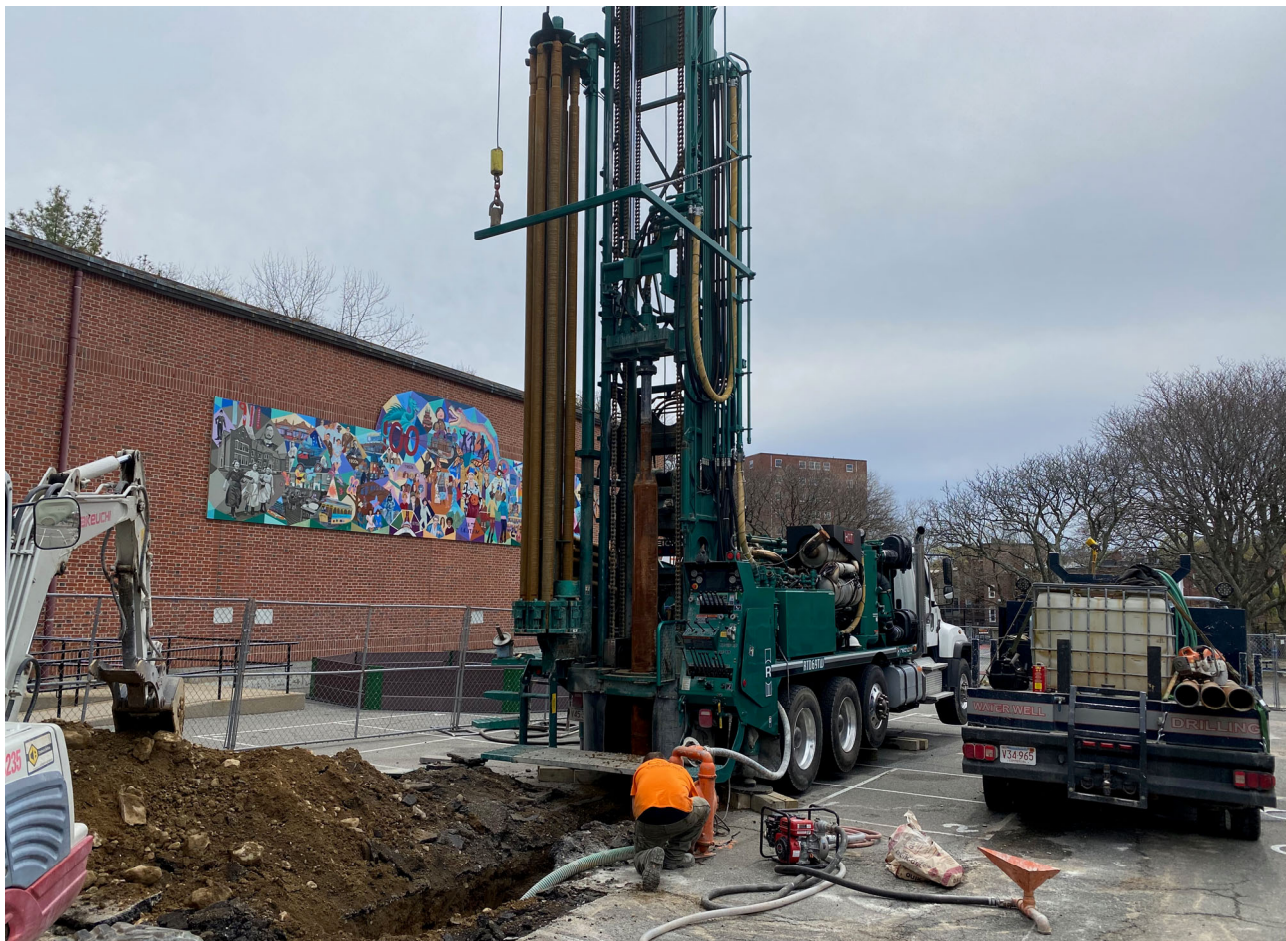
Installation of Test Geothermal Well
